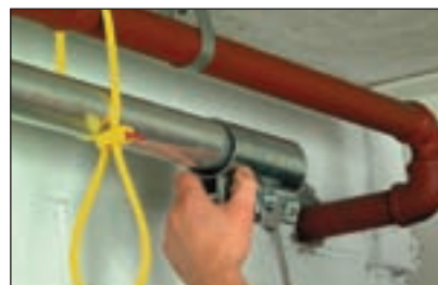
SpeedyTie® is particularly suited for temporary but safe bundling or fixing.
